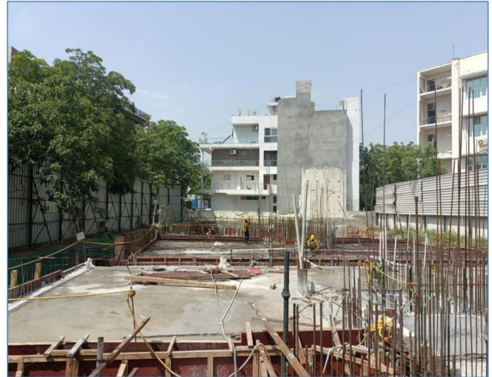
Plot Number 3613, 3615, 3617 & 3619 GF Slab WIP
