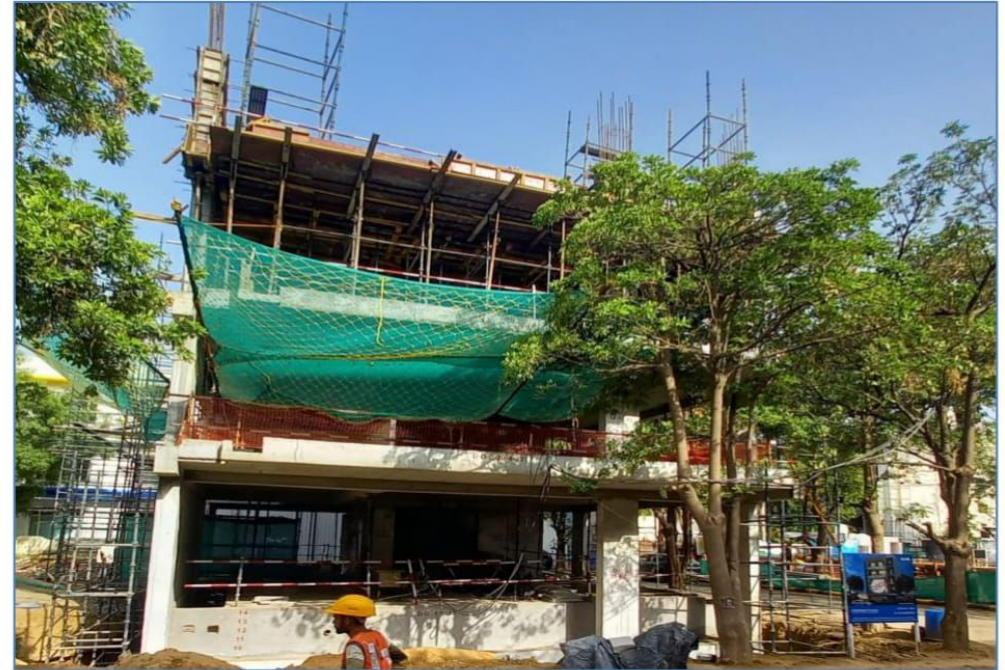
Plot Number 4814 3 rd Floor Slab Completed
