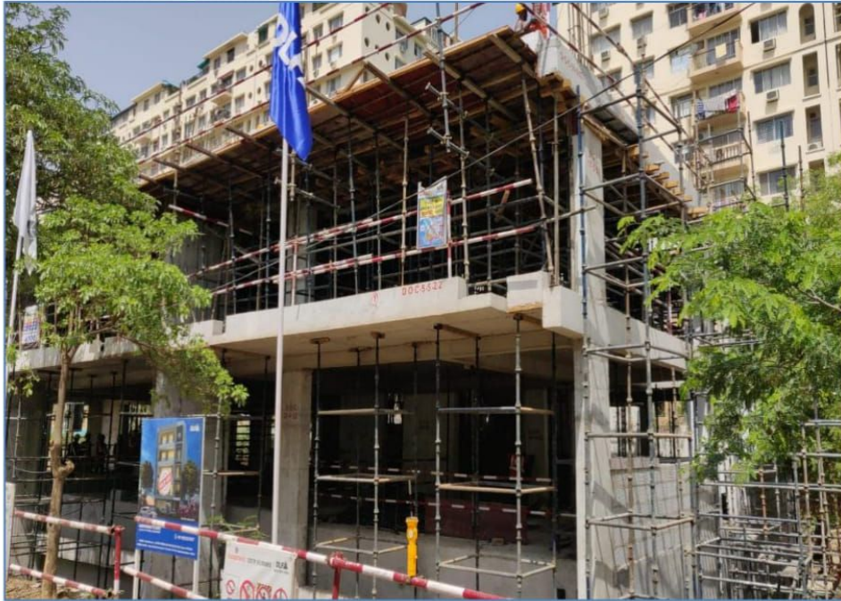
Plot Number 4813, 4815 & 4816 2 nd Floor Slab completed
