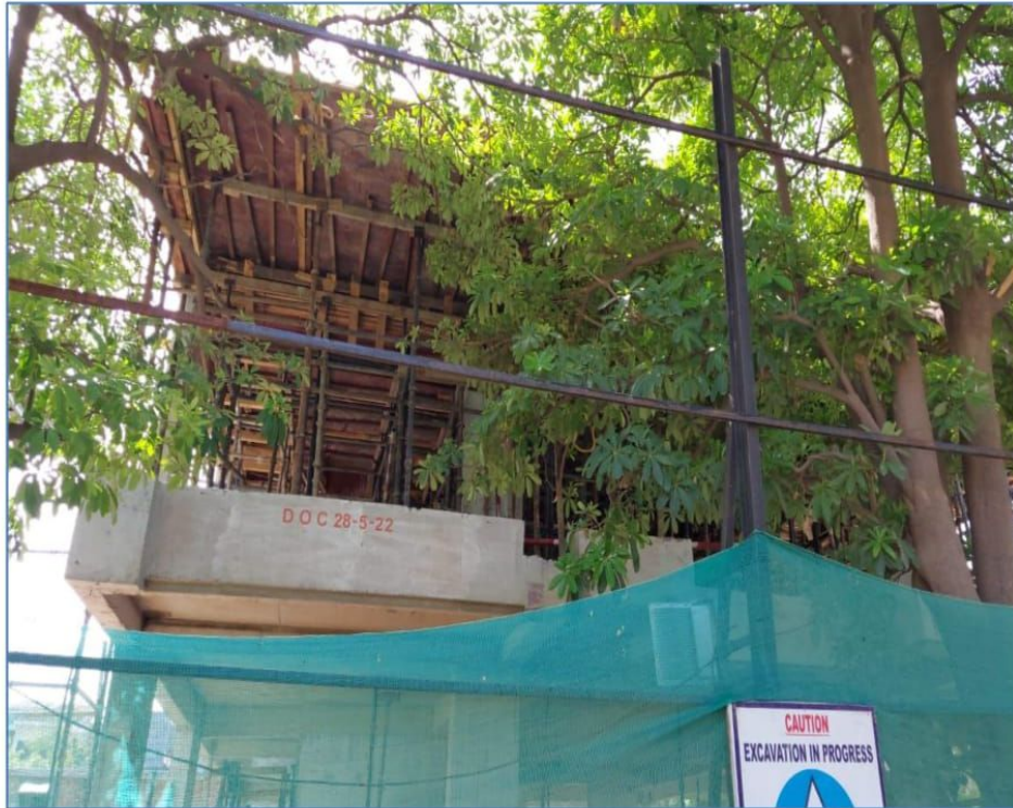
Plot Number 1031 2 nd Floor Slab Completed
