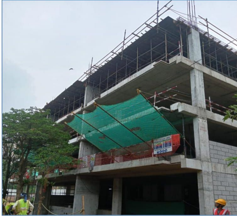
Plot Number 4813, 4815 & 4816 4 th Floor Slab WIP
