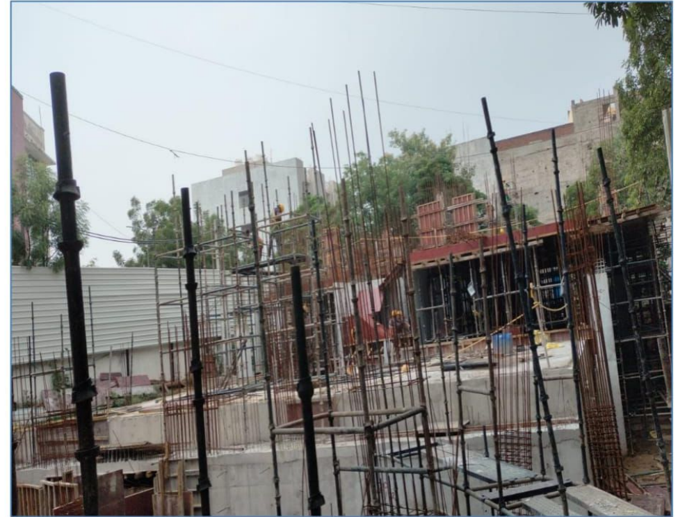
Plot Number 3613, 3615, 3617 & 3619 2 nd Floor Slab WIP
