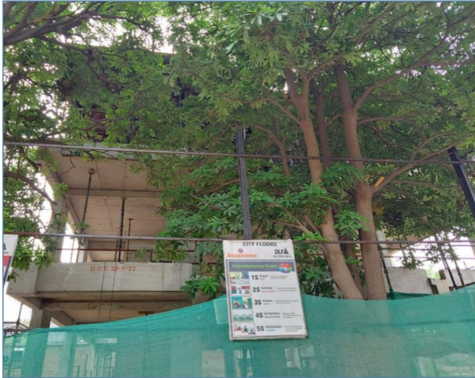
Plot Number 1031 3 rd Floor Slab Completed
