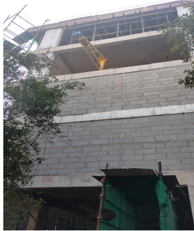
Plot Number 3613, 3615, 3617 & 3619 4 th Floor Slab WIP
