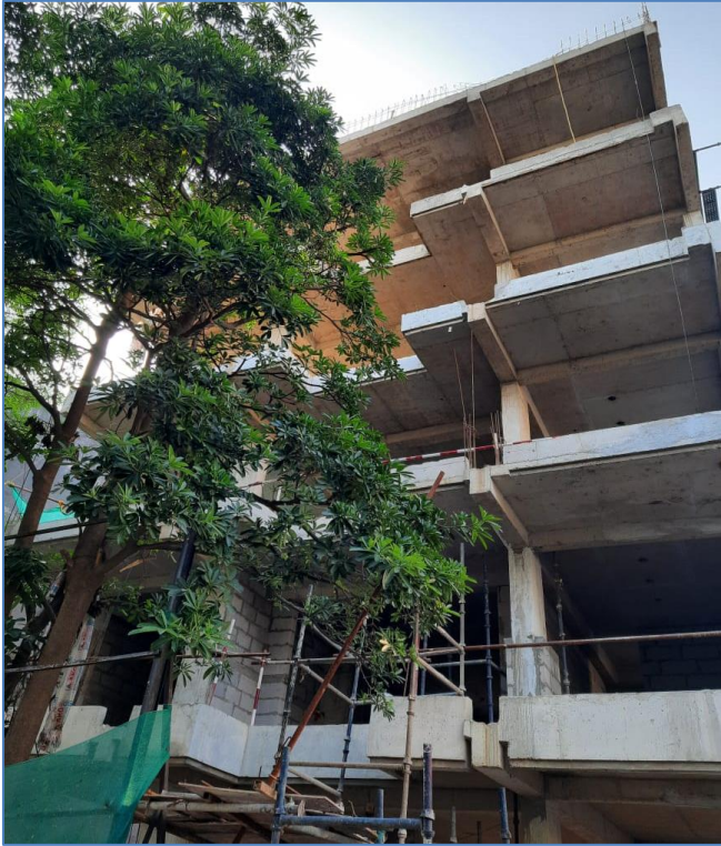
Plot Number 1031 Terrace Slab Completed. B/w & Plaster WIP
