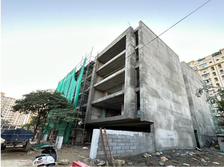
Plot Number 4813, 4815 & 4816: External plaster & finishing WIP
